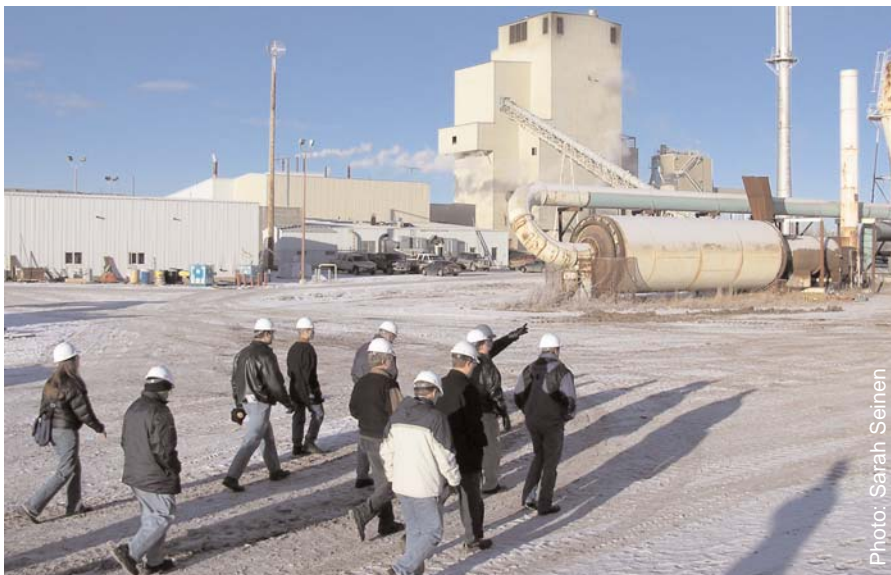
Recent field tour of biomass energy plant in Dapp, Alberta
